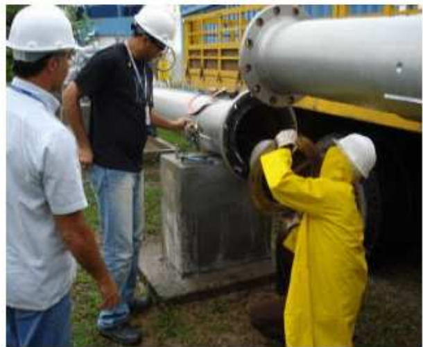
Photo I – Installation of the Magnetic Filter (6 Nov 2007)
