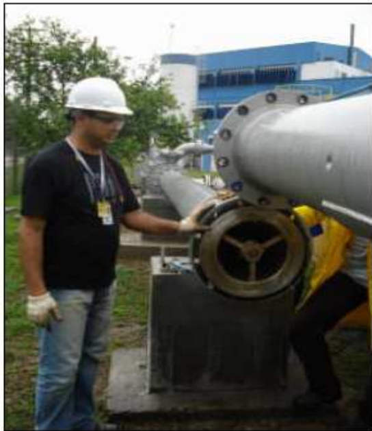
Photo F – Retrieval of Magnetic Filter (6 Nov 2007)
