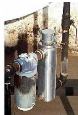
Above: Series 5000 Scrubber Rod with ferrous contamination from a diesel bulk fuel tank. Below: 5000 Scrubber installed inline before the traditional fuel filter
